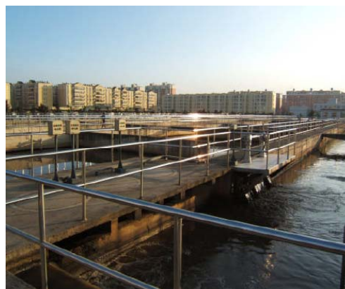
Biological treatment unit (A2O) WWTP No. 5
