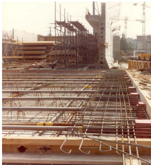
Construction of aeration tanks for biological treatment
