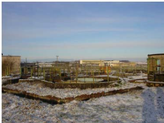
WWTP Telsiai before retrofit and expansion
