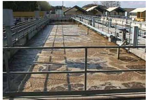
Activated sludge treatment unit and gravity filtration
