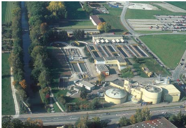
Aerial view of WWTP Kloten-Opfikon, Switzerland
