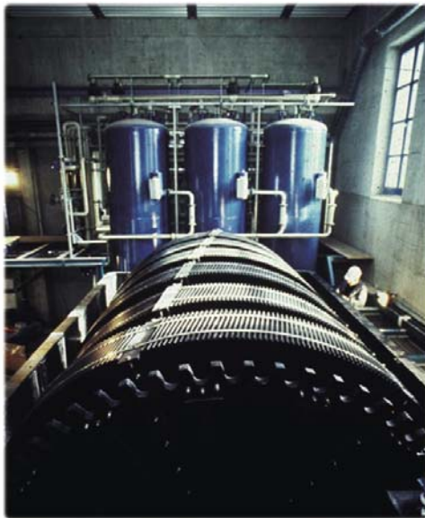
above: rotating disc filter for decomposition of carbon, in the background three activated carbon filter with 3 x 5m 3 volume and total 2550 kg carbon
