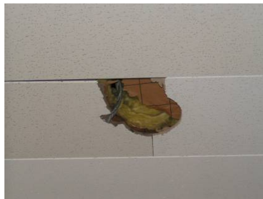
Asbestos: research and sampling under roofs
