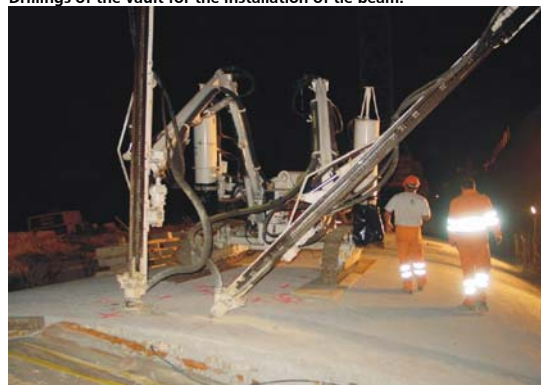
Drillings of the vault for the installation of tie beam.
