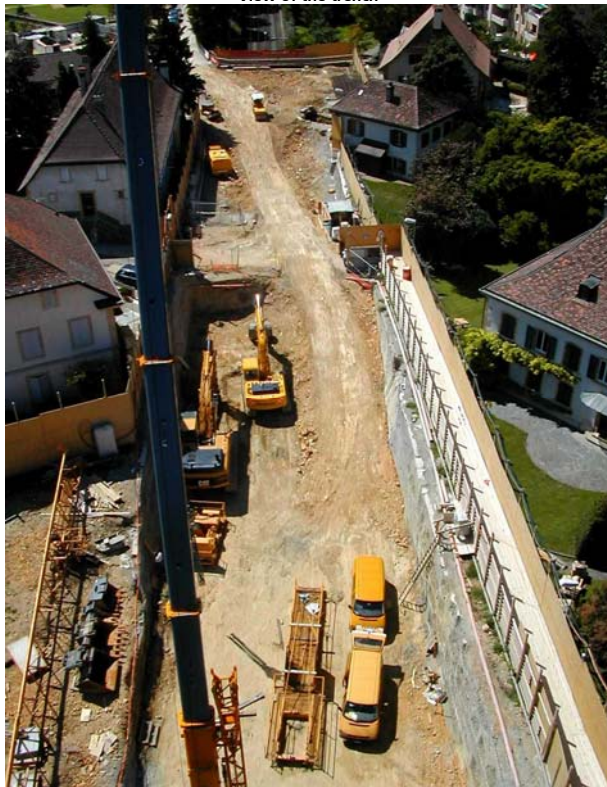
View of the trench
