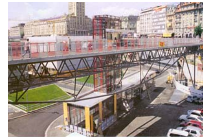
Place de l'Europe, bridge and lifts
