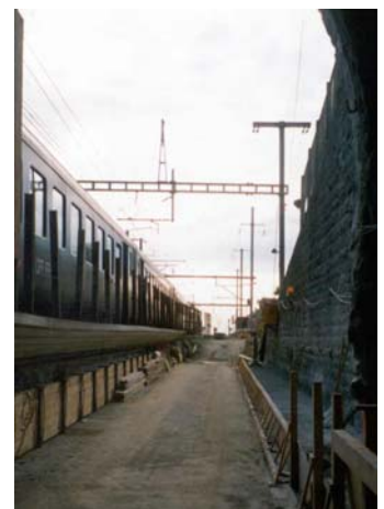
Lowering the foundation and installations towards the gate
