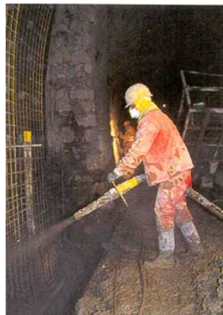
Rebuilt of a supporting wall with concrete
