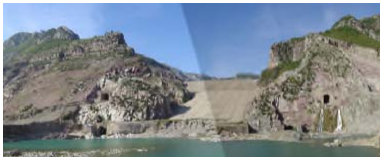
Downstream face of the Komani Dam
